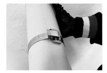
**7.** Press the band end downward between the ears with your thumb.
