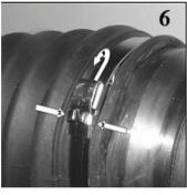
Complete clamp installation by tapping down the tail of the clamp against the buckle and then tapping down the buckle ears to hold the clamp tail. Remove excess band from the tool by lifting the locking pawl and removing the ratchet.
